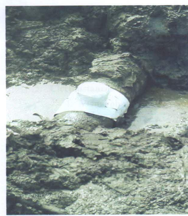
REPAIRED POINT – WRAPPED
