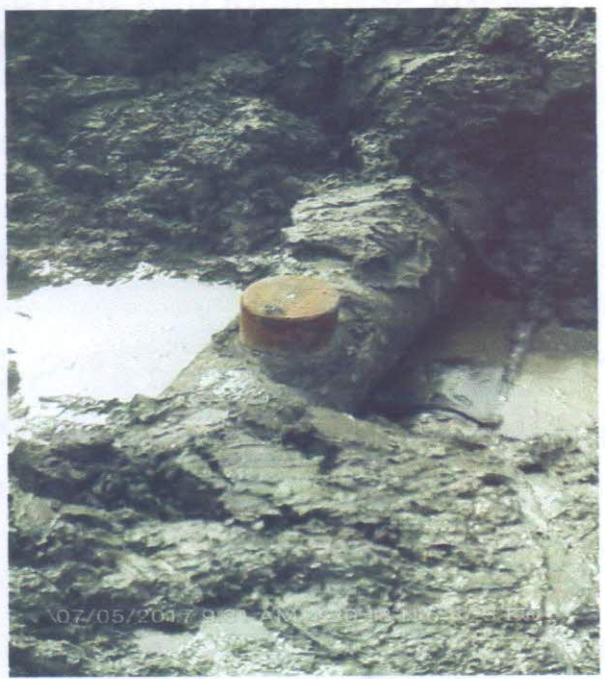
INTERFERENCE POINT- REPAIRED
